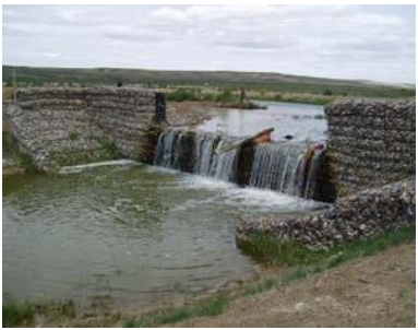
Gabion dams protection
