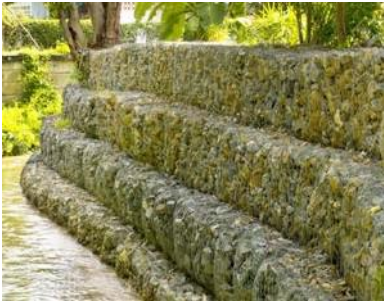
River bank protection
